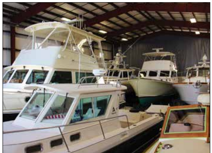
The 40,000-square-foot facility keeps the yard busy during the winter, providing climate controlled space storage and work.
